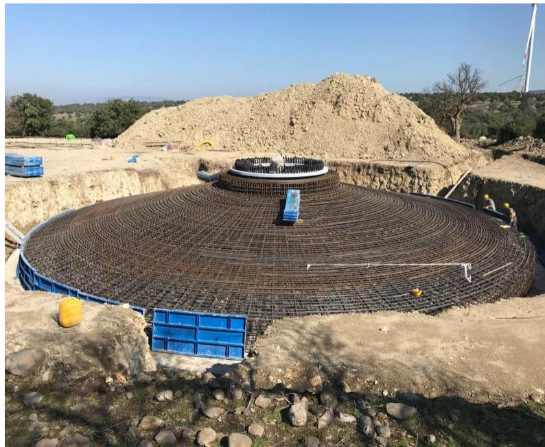
Figure 2. Wind turbine foundation.
