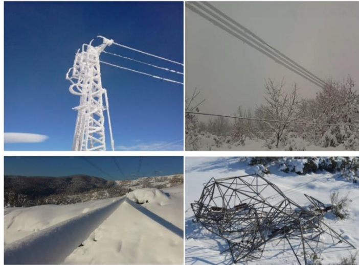
Figure 2. Damages are caused by snow load and icing in Turkey (EKOL, 2019).
