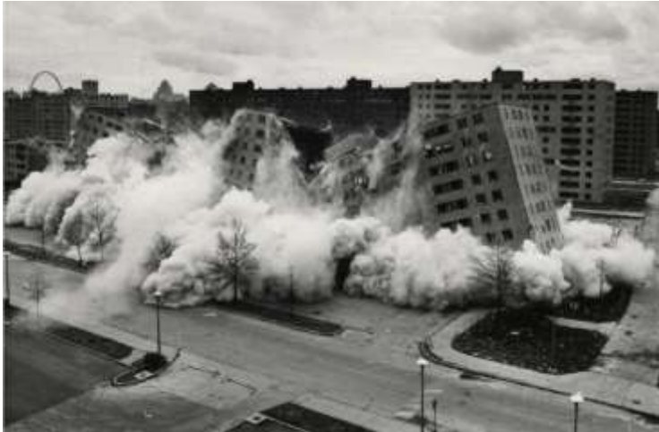
figure 14: 38 Minoru Yamasaki - Pruitt-Igoe, Missouri, 1972 (demolition).
